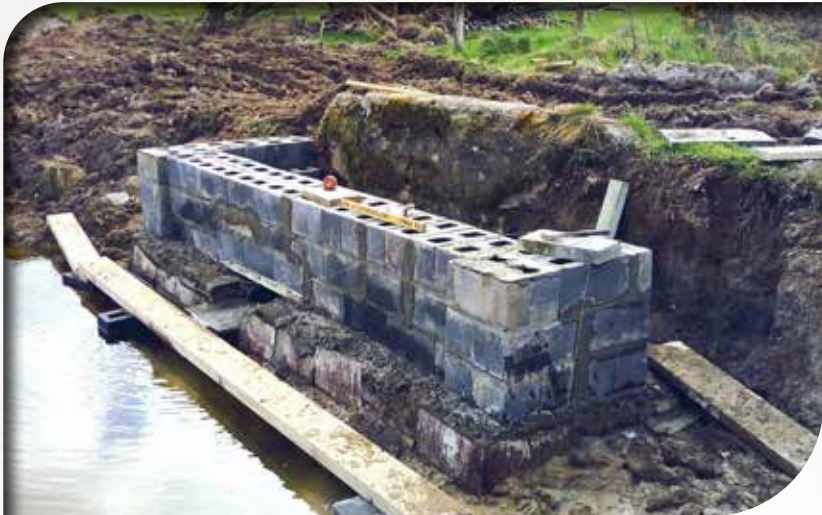
several layers of cement block to 1.5 metres above ground level
