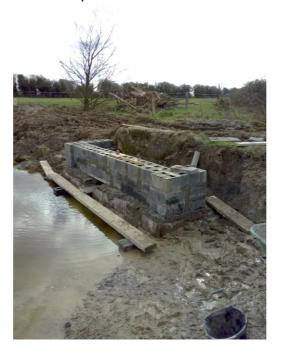
• From that point onwards use the cavity blocks - two rows placed side by side.
